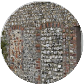
Red brick arch detail in a former doorway
