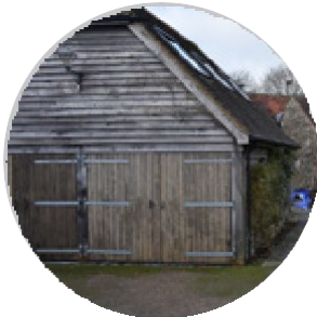
Timber weatherboards
