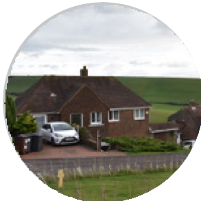
Combination gabled and hipped roof
