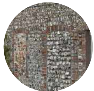
Red brick arch detail in a former doorway
