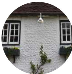
White painted flint facade with timber casement windows
