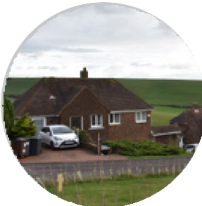
Combination gabled and hipped roof
