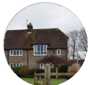
Clay tiled gabled roof
