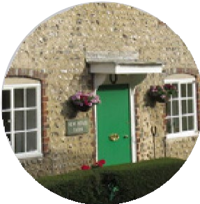
Flat roofed open porch
