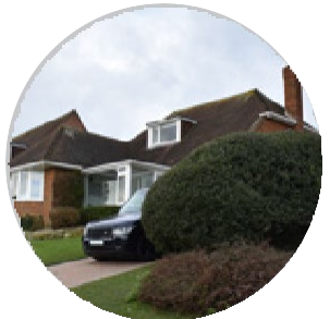
Hipped roof with dormer
